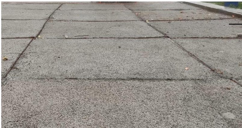
Pervious concrete pavement infiltrating stormwater without runoff generation
