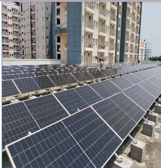
Solar PV panel installation in Progress.
