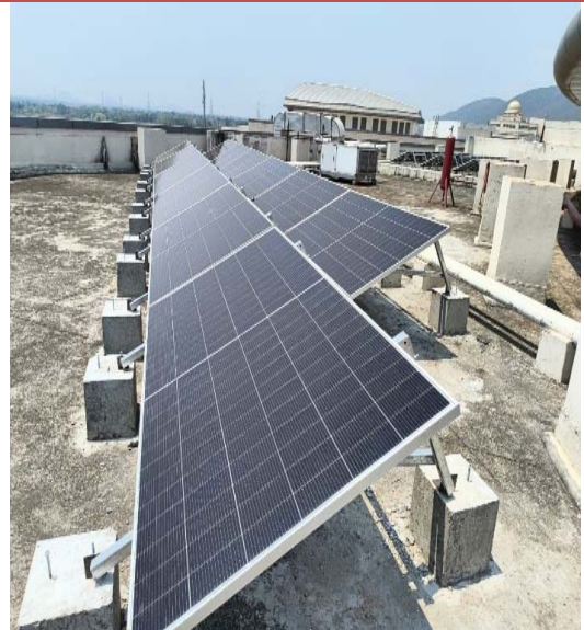
Solar PV panel installation in Progress.
